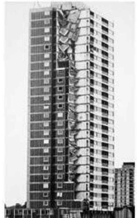
Figure 3 Progressive Collapse - Ronan Point, London, 1968
